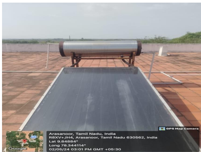
SOLAR WATER HEATER ON THE ROOF TOP OF MECHANICAL BLOCK
